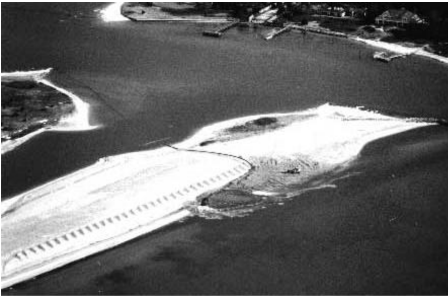
Dredging in action: West Bay sand stabilizes Dead Neck.
