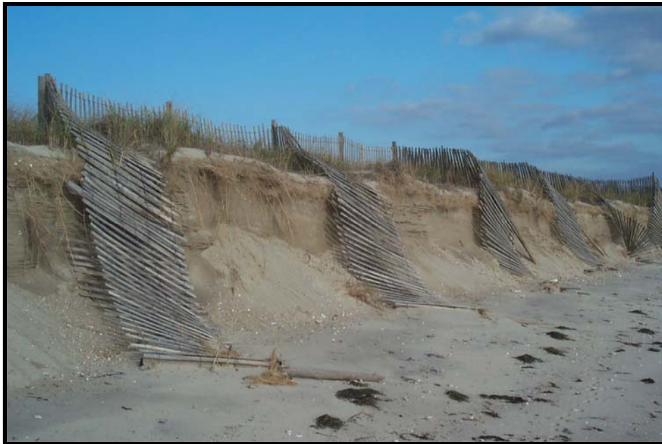
Figure 4. At the time of the November 2002 shoreline survey of Dead Neck, sand fencing set-up in the nourishment area had begun to fail due to erosion of the beach fill.
